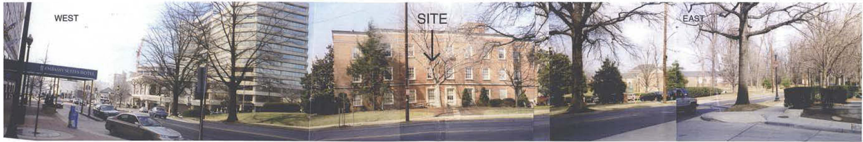
1. VIEW OF THE SITE FROM MILITARY ROAD
